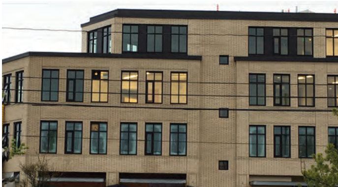
Encouraged Materials: The use of brick, high quality “punched” (recessed) windows, metal awnings and cornices shown above both relate to traditional neighborhood materials and contribute to a feeling of lasting durability
