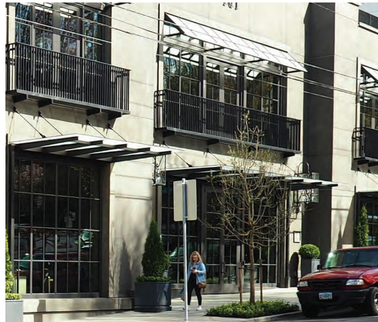
Awnings, balconies and storefront windows help break up larger facades and relate to a more human scale. NW Portland (Image: M. Molinaro)
